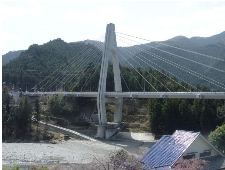
Fig. 2-5. Okutama Cable-Stayed Bridge: TMD for suppression of Vortex-Induced Vibration
